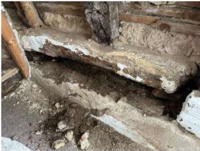
severely rotted sole plate
