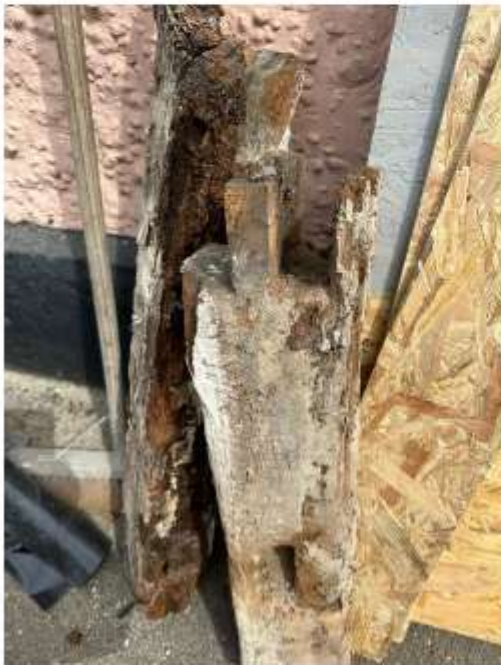
rotted sections of studs
