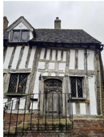
The images left show the street elevation defective panels marked with red crosses, the panels removed, and the finished work.
