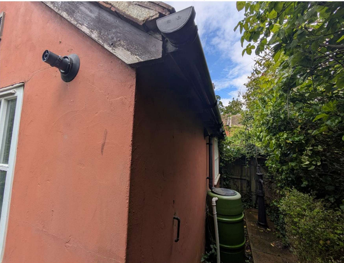
Photo 3 Side of the existing extension
