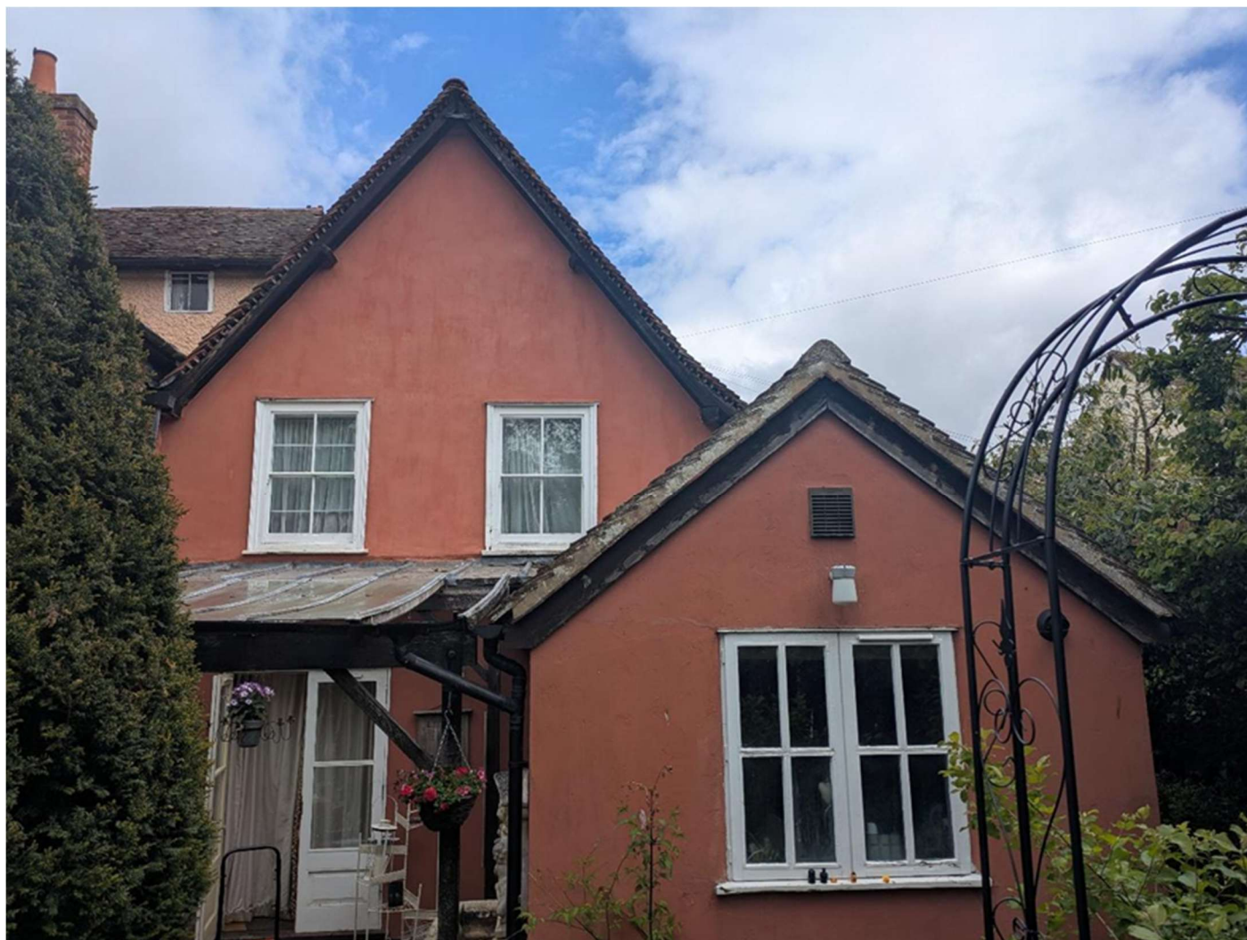
Photo 1 Existing covered area and pitched roof extension
