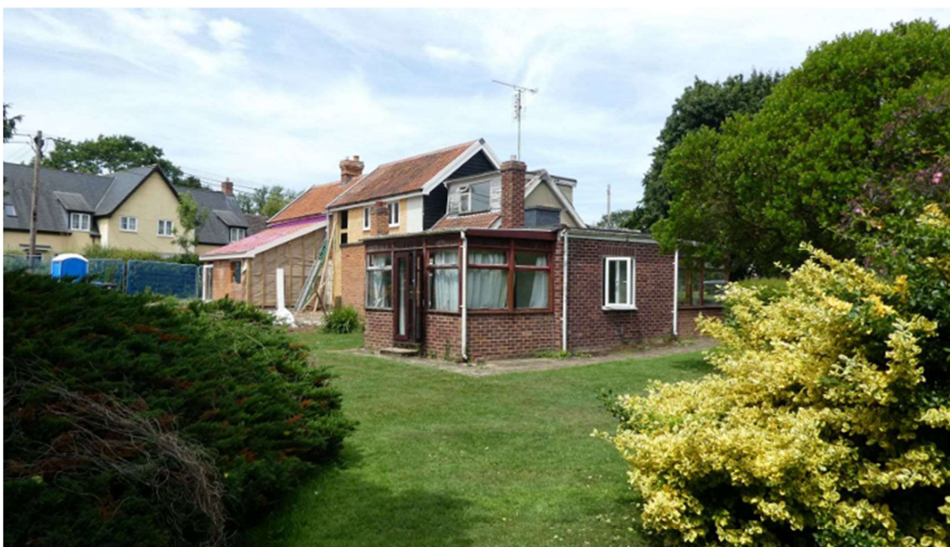
Fig.5 - The existing house looking westward with the recently extensively refurbished neighbouring property (Glenholme) behind. The houses in the background are the other side of the Brent Eleigh Road and are significantly higher.
