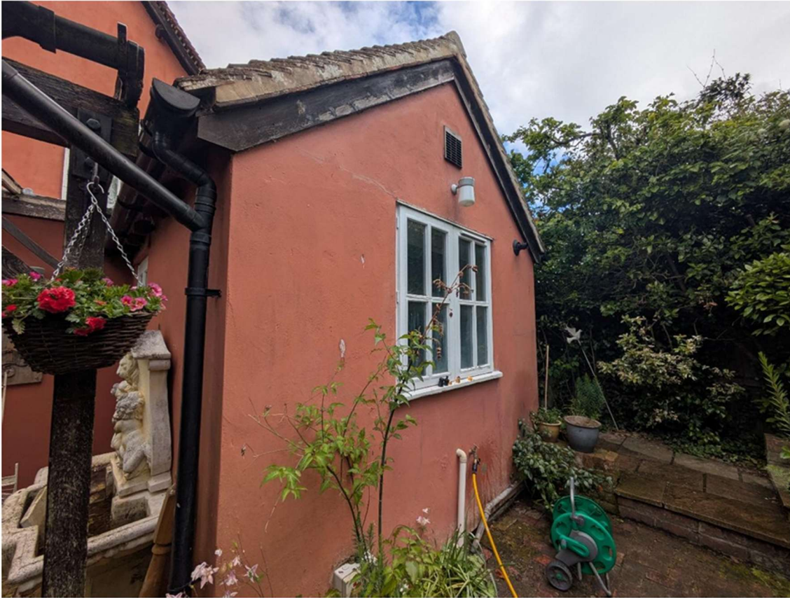
Photo 2 Pitched roof gable end where a small extension is proposed
