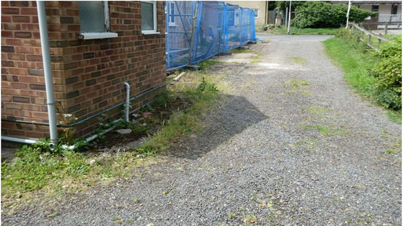
Fig.2 - The existing permeable granular finished drive to Poultry House coming off Brent Eleigh Road
