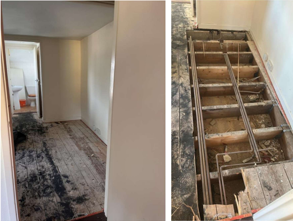
Photos showing position of proposed new staircase location and modern floor joists to be removed / modified to accept new staircase.
