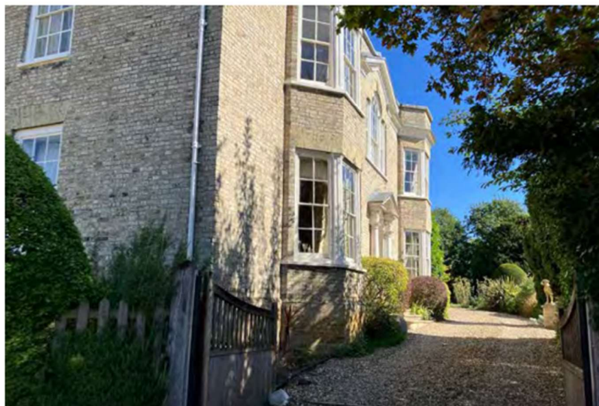
Above: Principal entrance to the site from Lady Street
