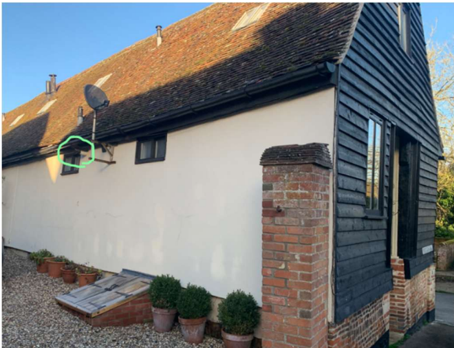
Current flue exit location
